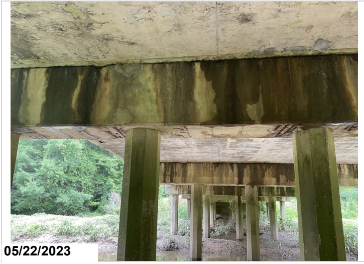
Bent 3 bottom of cap has spalls with exposed rebar.
