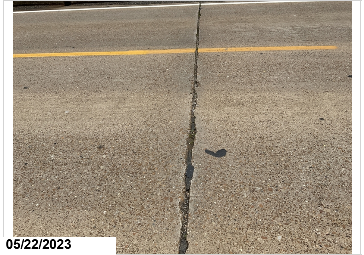
Bent 4 joint seal has lost bond.
