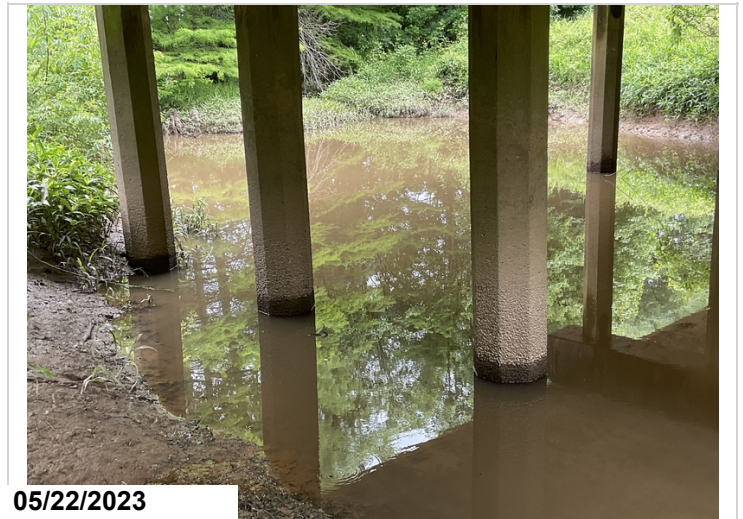
Bent 4 pile have abrasion.
