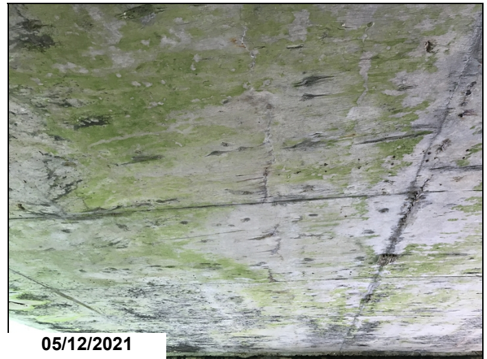
Span 2 cracking reflecting from top side of deck
