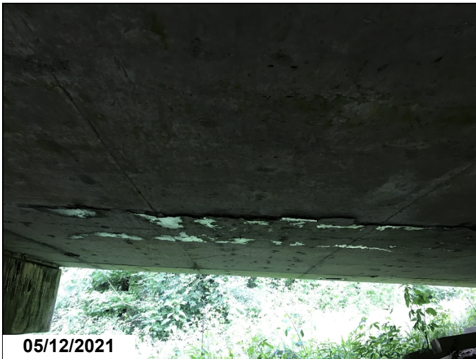
Span 8 soffit on left lane has large delam with cracking and staining.
