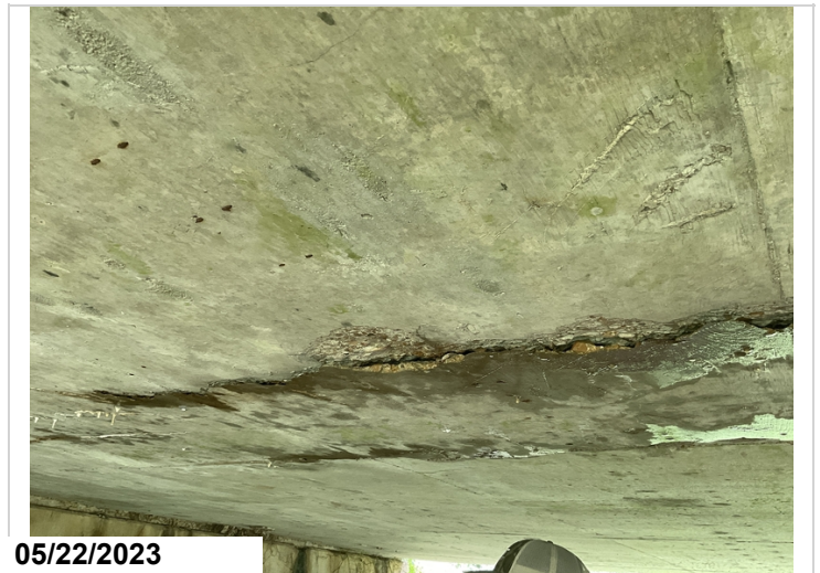
Span 7 large soffit delam.
