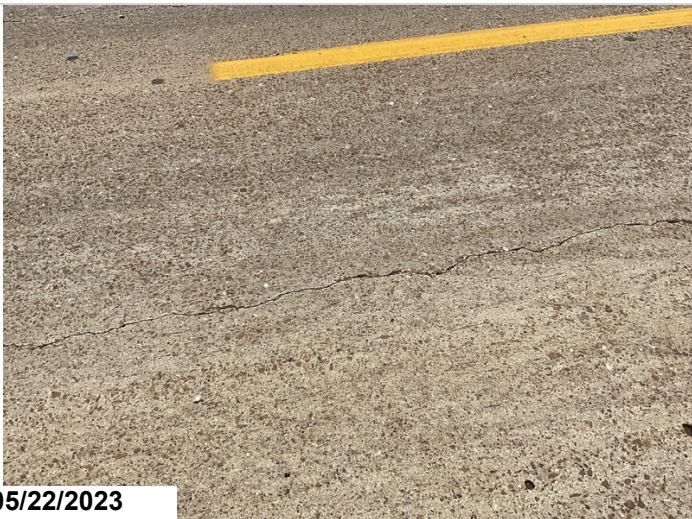
Span 1 deck cracking.
