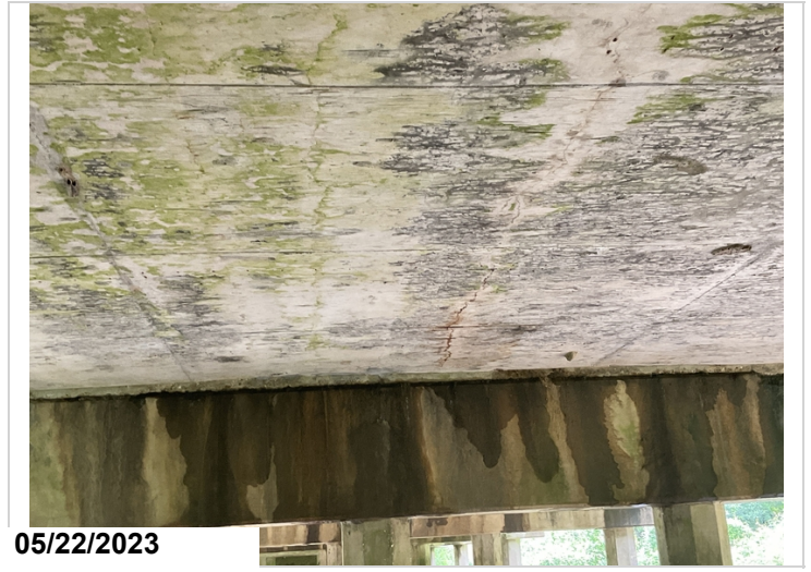
Span 2 soffit has large cracks with staining.
