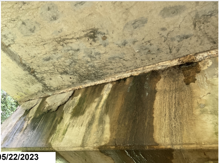
Bent 7 cap back has spalls and delams.
