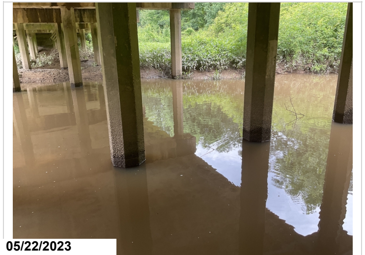
Bent 3 Pile have abrasion.
