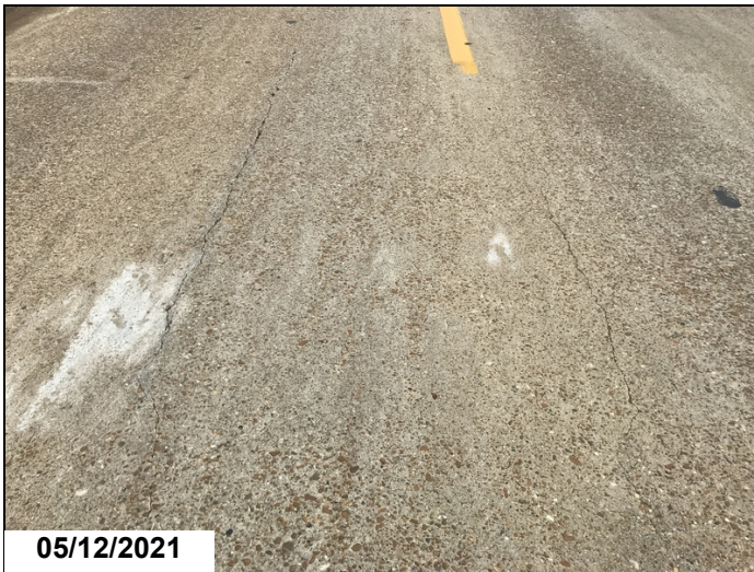
Span 2 large unsealed crack that reflect to soffit.
