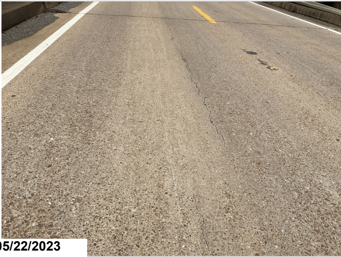
Span 6 deck cracking.
