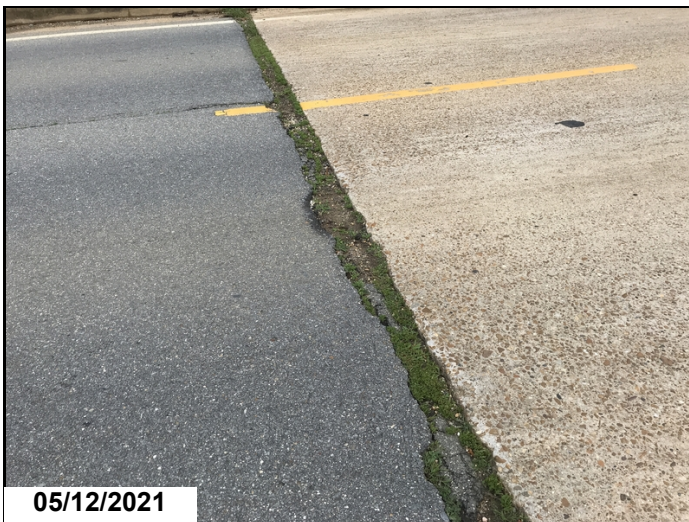
Bent 1 and roadway approach, Joint filled with debris.
