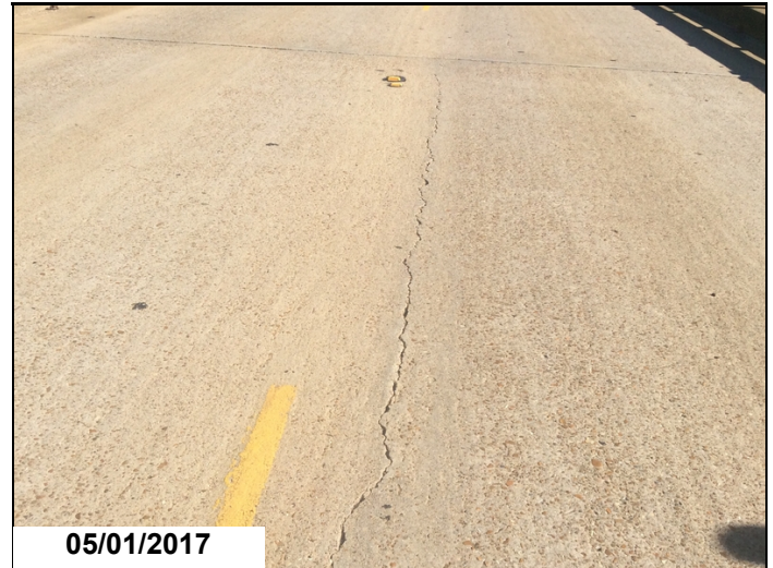
Large crack on span 4 near centerline but common on spans 1,3,4,5 & 6
